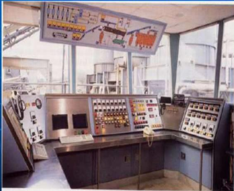
Photograph 12.8 – A modern drum mix plant control room (Photograph reproduced by kind permission of Redland Aggregates Limited)
