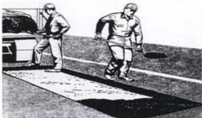
Backfilling Hole with Plant Mix
