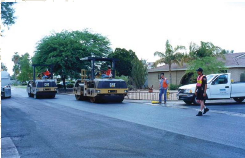
Photograph 13.3 – A traditional deadweight roller
