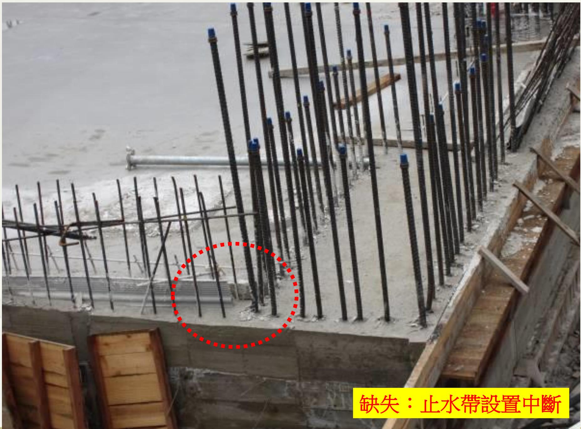
缺失：止水帶設置中斷
