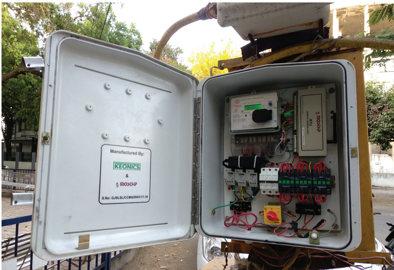
Figure 3: Central Control Monitoring System
