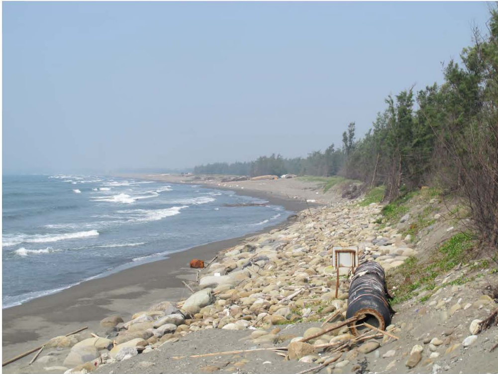
Photo 15. Eroded area downcoast of groins.
