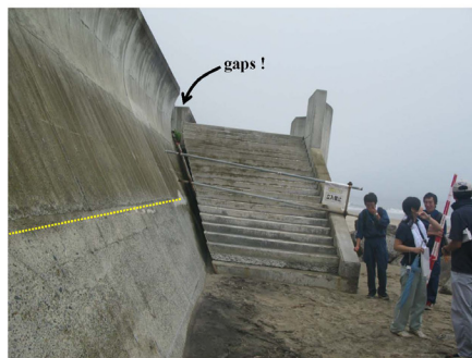
Figure 6. Damaged stairs looking the front (July 9, 2009).
