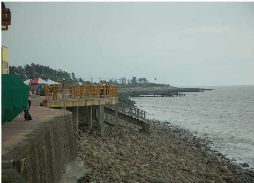
Fig. 4. Severely eroded beach with exposure of gravel bed (September 1, 2012).
