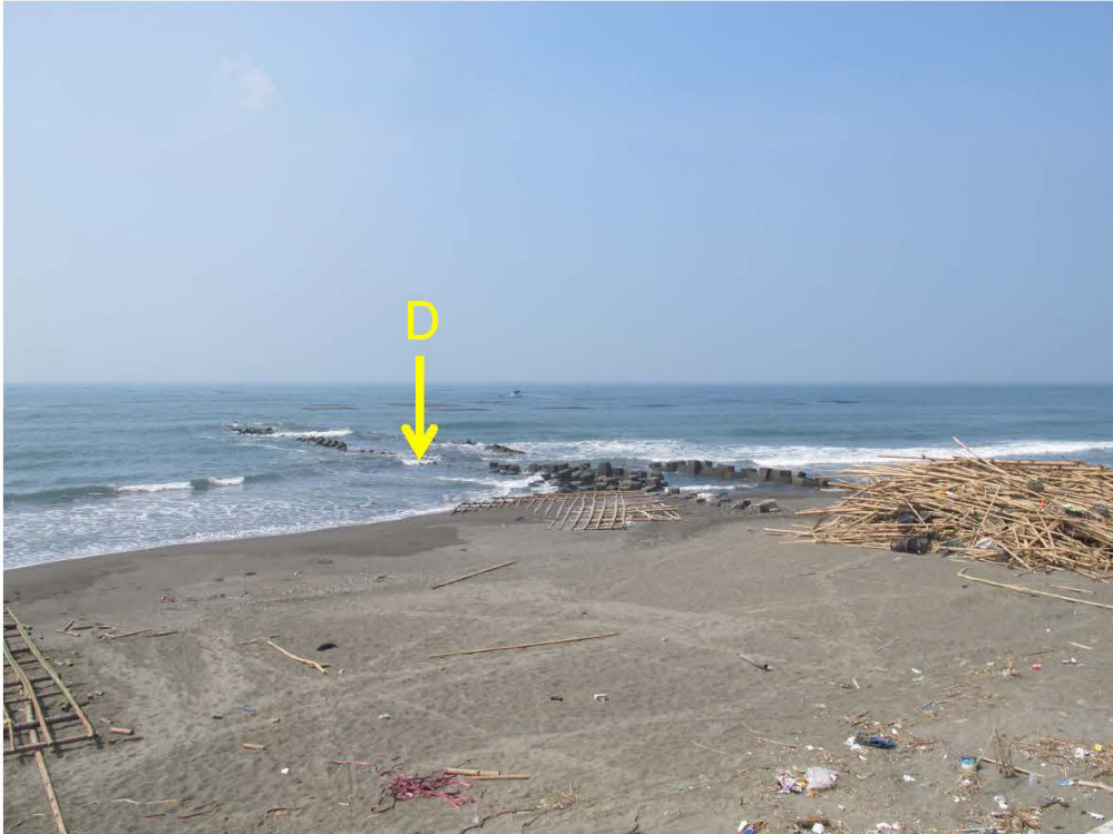
Photo 13. Enlarged view of groin at north end of beach.
