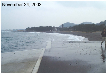
Figure 15. Wave overtopping to the corner of the seawall (November 24, 2002).
