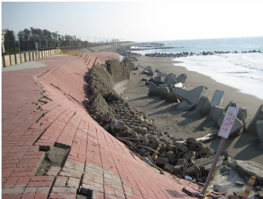
Fig. 2. Collapsed seawall and concrete armor units (January 26, 2011).
