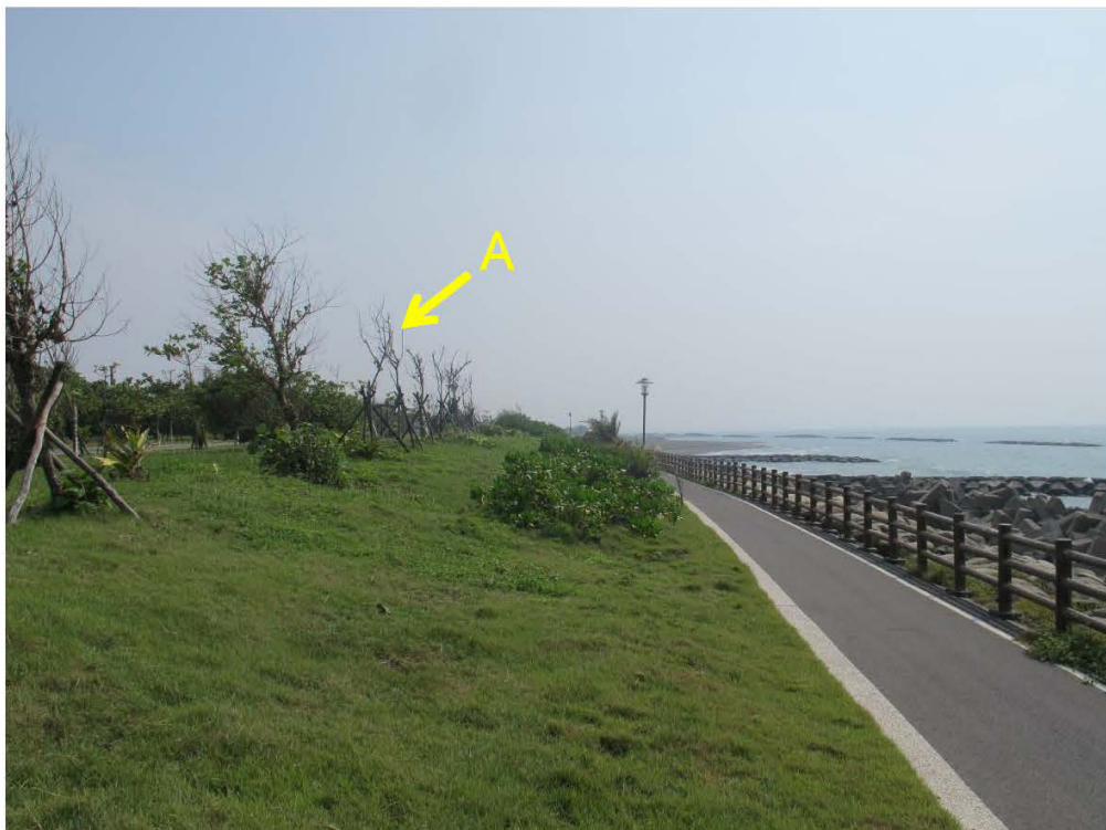
Photo 6. Coastal dike with gentle slope and vegetation.
