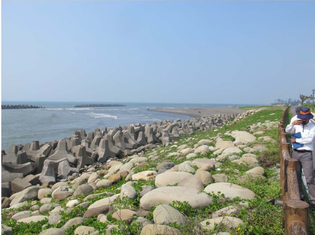
Photo 5. Large boulders and concrete blocks to protect coastline.
