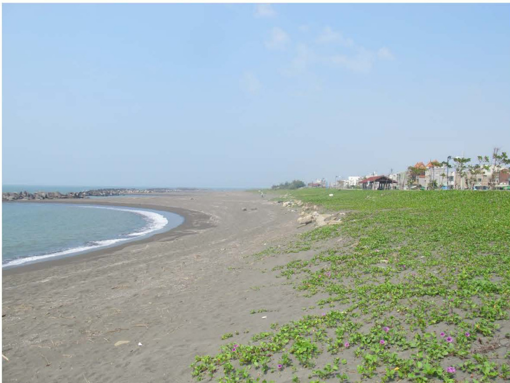
Photo 2. Cuspate foreland formed by depositional effect of detached breakwaters.
