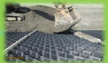
框內土方回填
